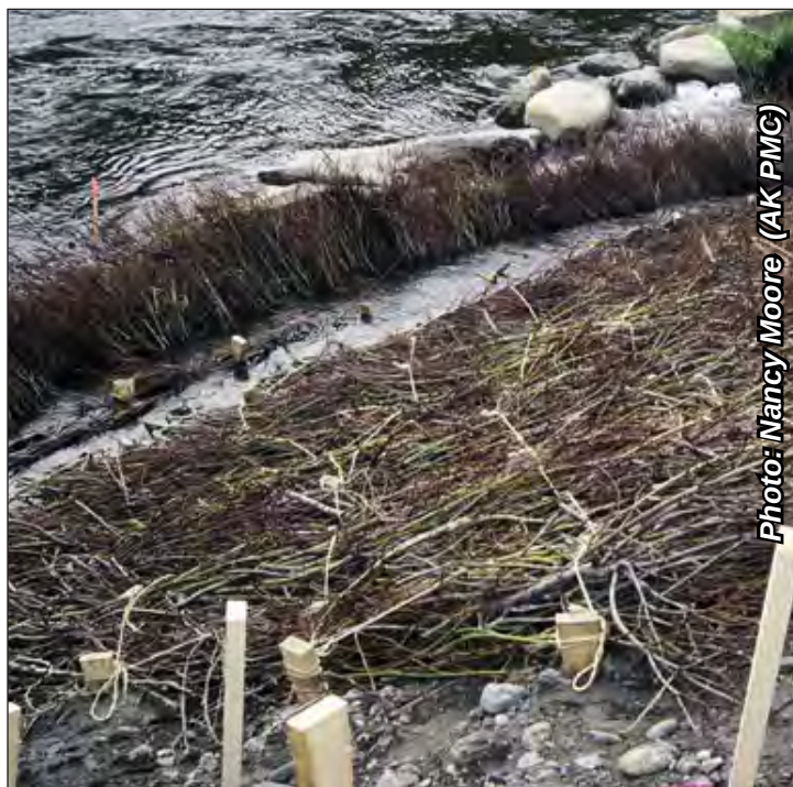
Figure 18: Willow cuttings were used to re-establish vegetative cover on the banks of the Kenai River
