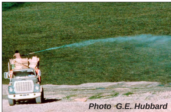
Figure 11: A truck-mounted hydroseeder applies a seed mixture
