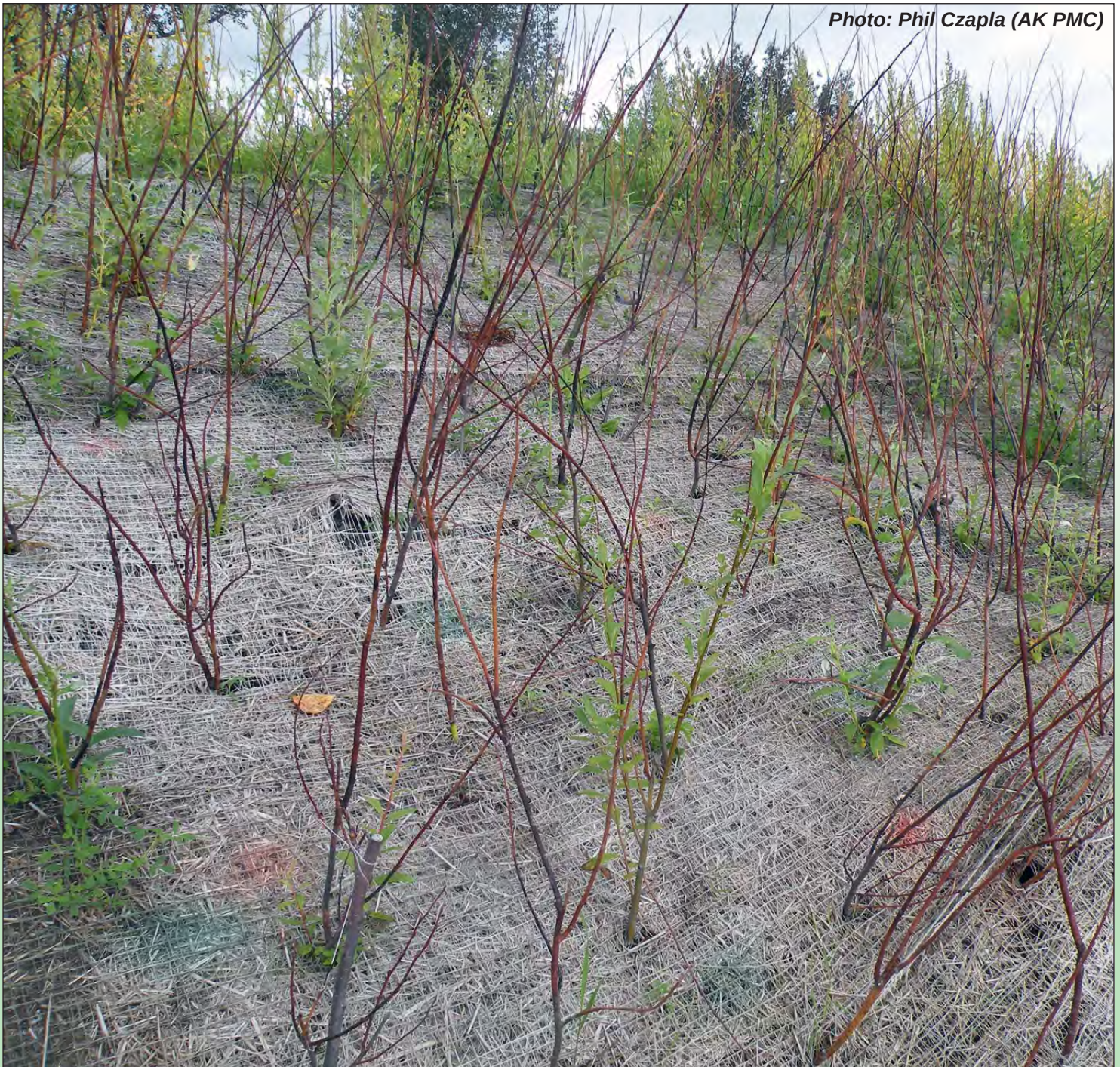
Figure 19: Erosion Control matting can stabilize a cut slope while seed or transplants become established
