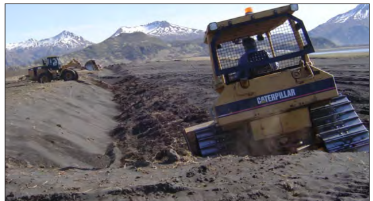
Heavy equipment used to spread topsoil - May, 2006
