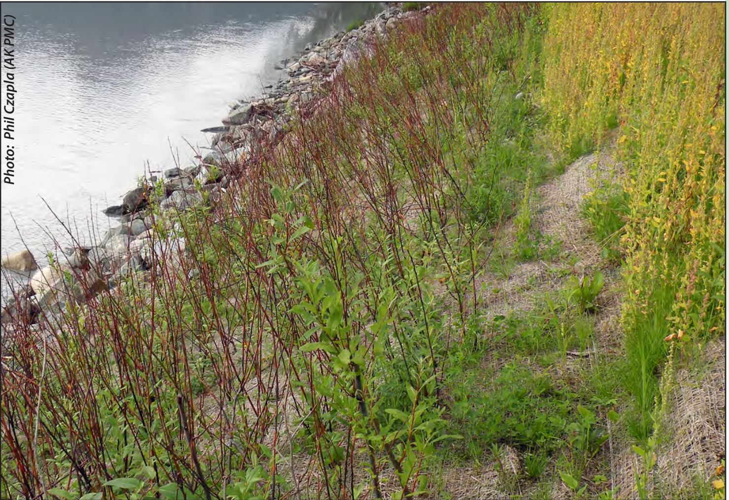
Erosion control fabric supporting willow stakes and seeded plants, along the banks of the Matanuska River
