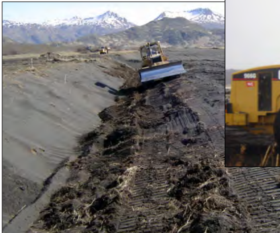
Spreading charged overburden - May, 2006
