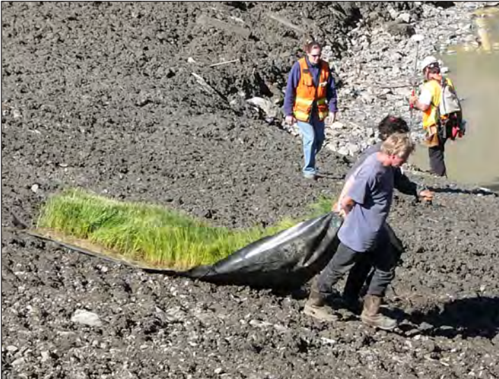
Heavy plastic sheeting facilitates on-site transport of the vegetation mats
