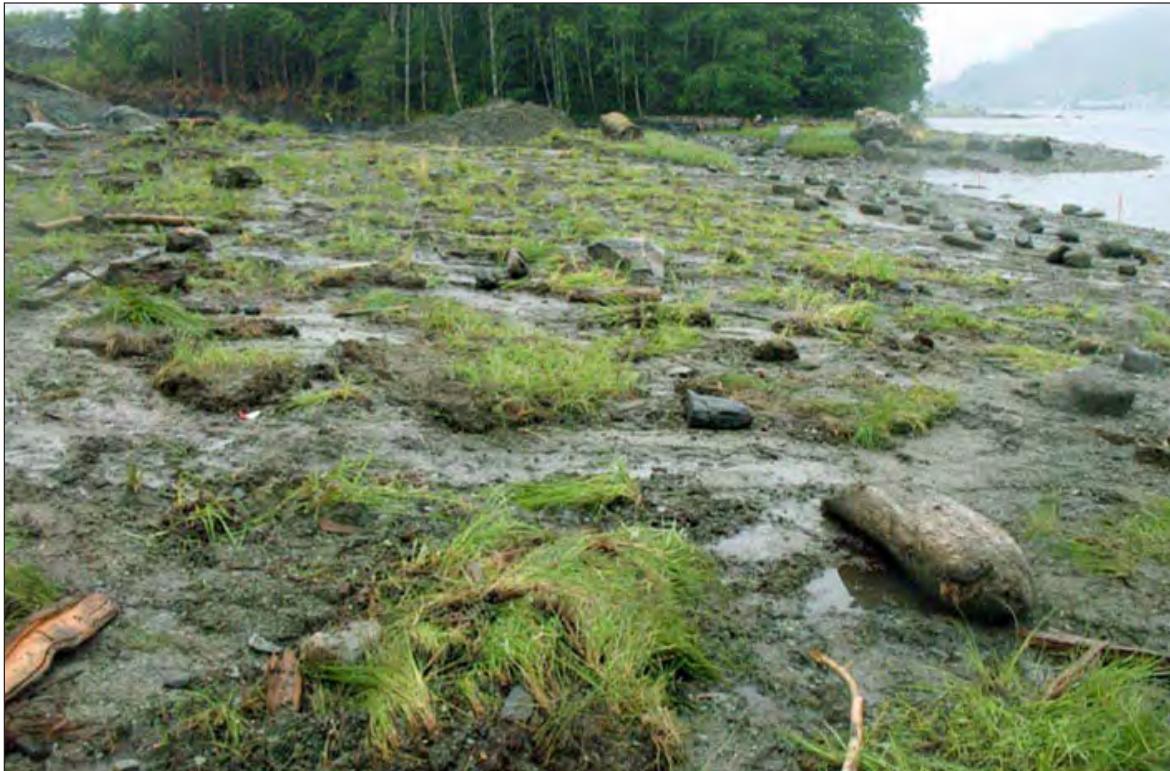
Clumps of sod deposited near an estuary to promote quick vegetation establishment
