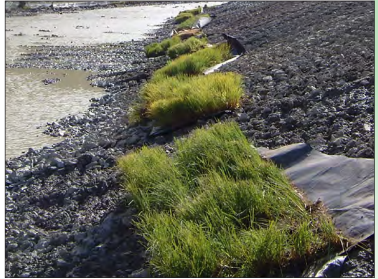
A line of vegetation mats, ready for placement
