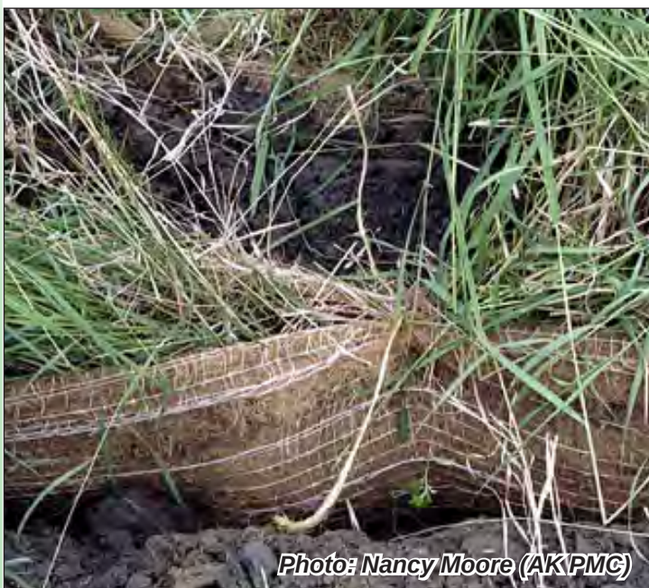
A prepared grass roll, consisting of sod clumps wrapped in an biodegradable fabric, with slits cut in the top for the shoots
