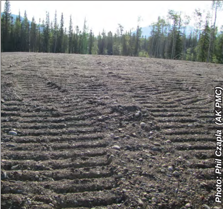
Surface imprinting accomplished using the 'track-walking' technique
