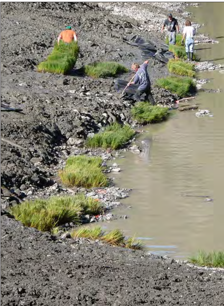
Vegetation mats being installed along the waters edge
