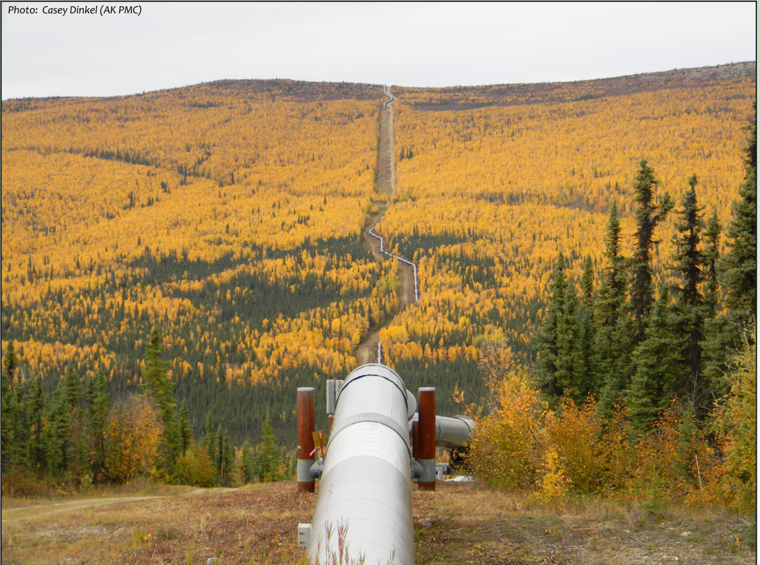
The Trans-Alaska Pipeline winds through mixed hardwood and spruce forest in Interior Alaska.
