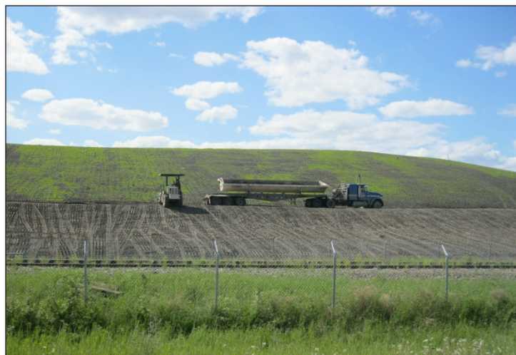
Site recontoured before topsoil placement - mid June, 2010
