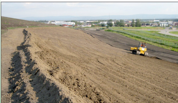
Salvaged topsoil was applied in a 6" layer all over the site.
