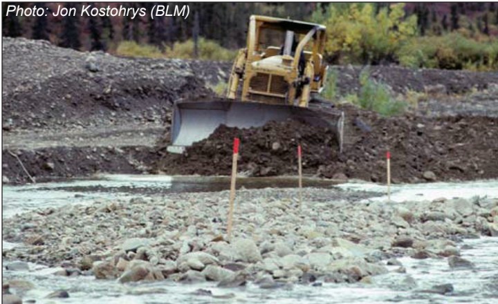
The initial step in reclamation was to fill the settling ponds using the material from the surrounding tailings piles.
