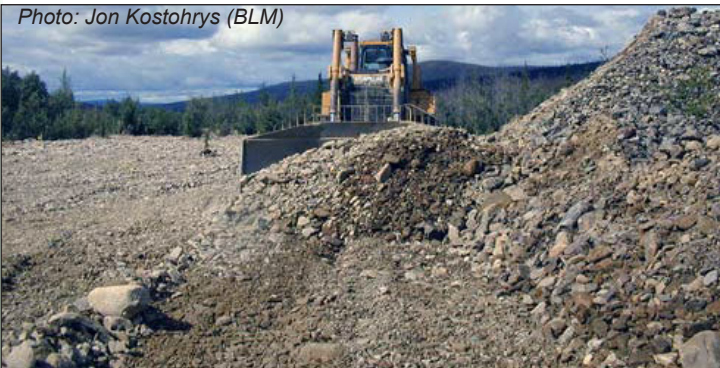
After filling the ponds, the bulldozer then graded the floodplain as flat as possible.
