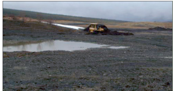
Dozer spreading organic soil during site preparation phase - June, 2003
