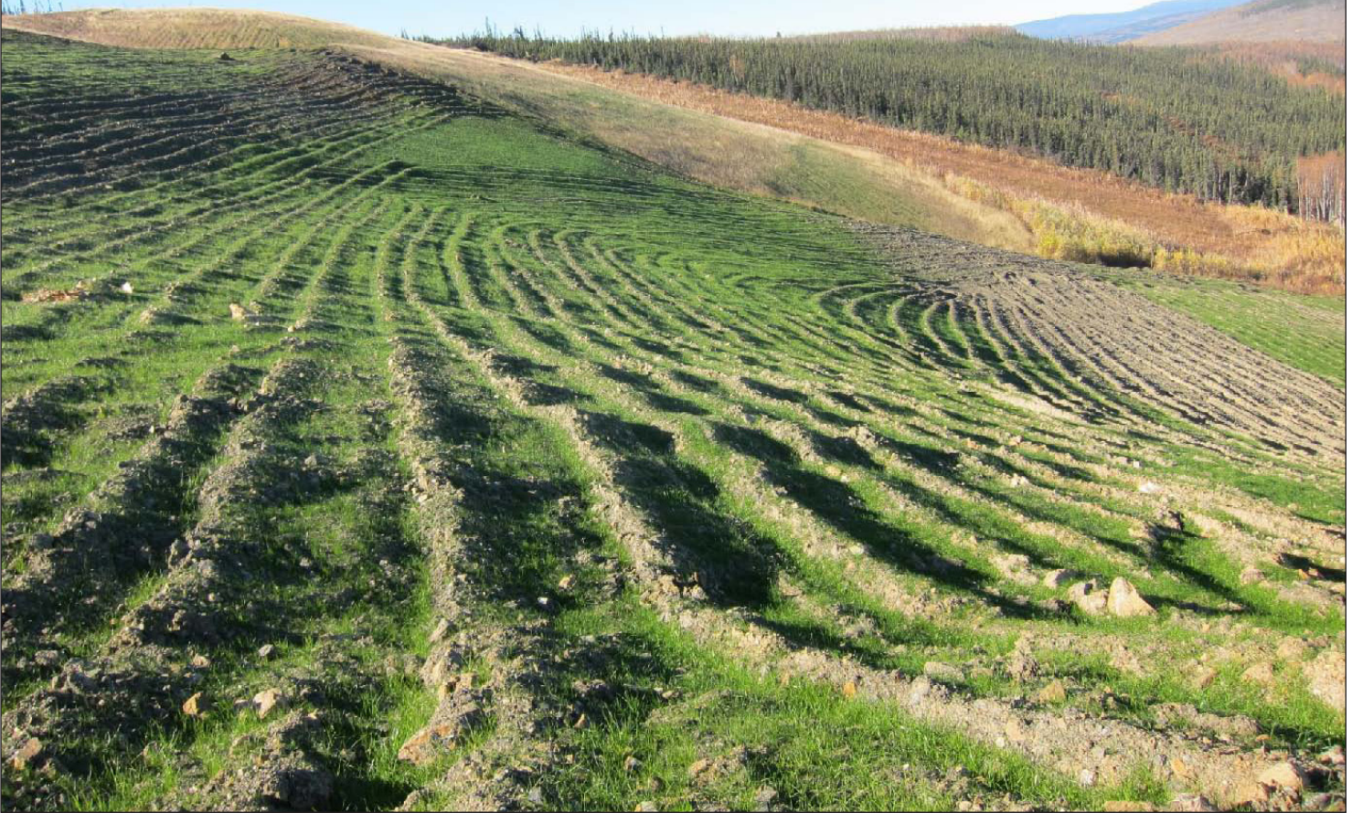
North Shepard dump - mid September, 2010 (seeded mid-August, 2010). Note furrows along horizontal contour of slope.
