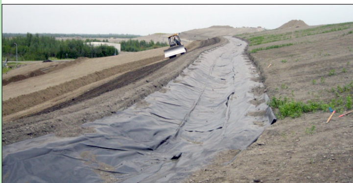
A rubber liner was placed along the length of the ditch in late June, 2010.
