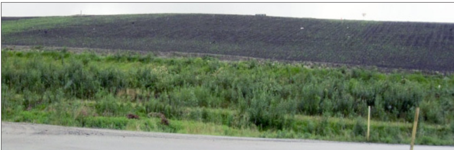
Two feet of N-Viro treated sludge was deposited on cell C/D - early June, 2010
