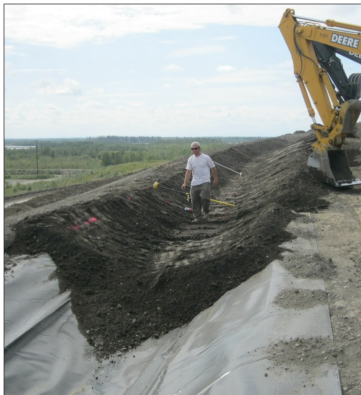
The ditch was filled in a three step process: 6" of gravel was placed over the rubber liner, followed by 18" of silt, and then capped with 6" of topsoil in early July, 2010.
