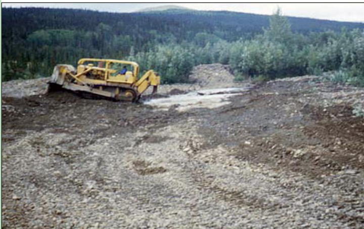
The bulldozer constructed the channel using short, almost level grading to deepen the pilot channel.
