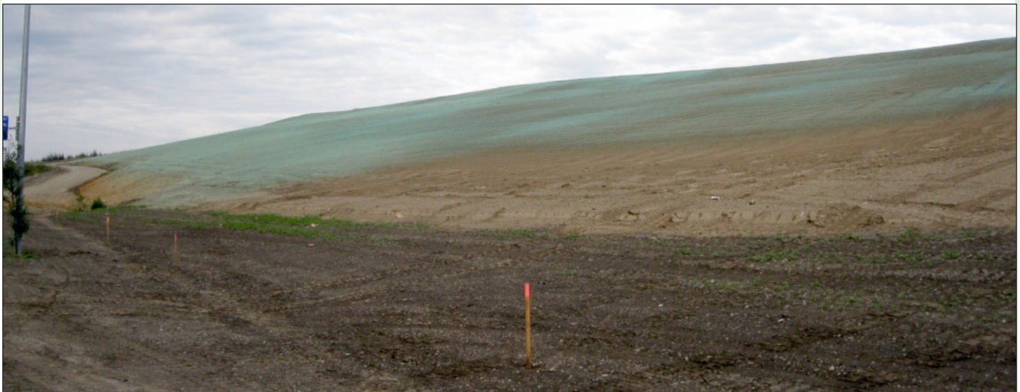
A hydro-mulch application of Eco-Fibre / Plus with tackifier was lightly sprayed over the area after drill seeding in mid July, 2010.
