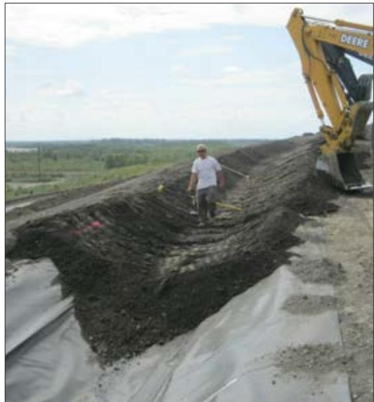
The ditch was filled in a three step process: 6" of gravel was placed over the rubber liner, followed by 18" of silt, and then capped with 6" of topsoil in early July, 2010.
