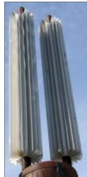
The Trans-Alaska Pipeline system uses ammonia driven "heat pipes" to ensure that permafrost underground remains frozen.
