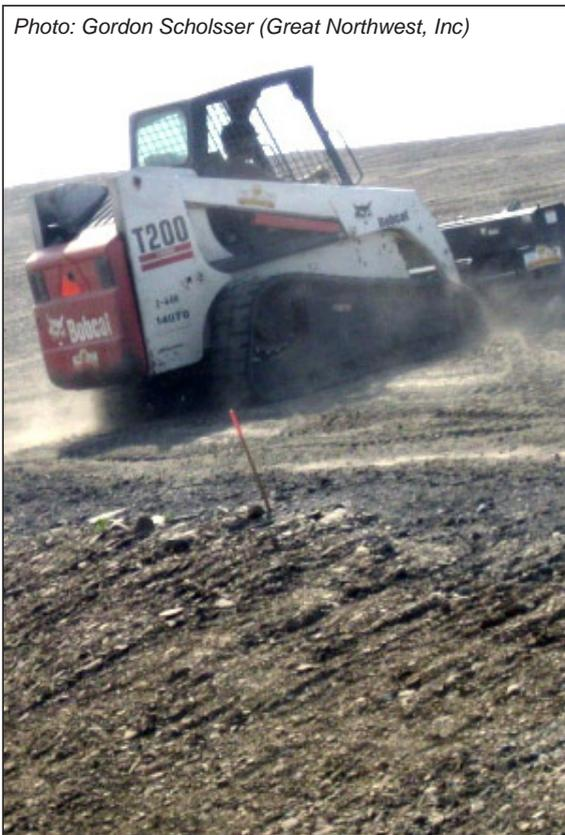
If operating on a slope, tracked vehicles should be driven up and down to the slope such that the cleat marks left after track-walking are roughly perpendicular to the slope
