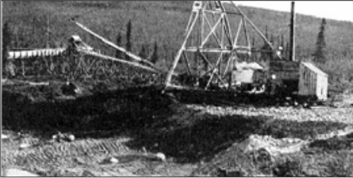
Drag-line used by a placer mining operation on Nome Creek in the early part of the 20th century.
