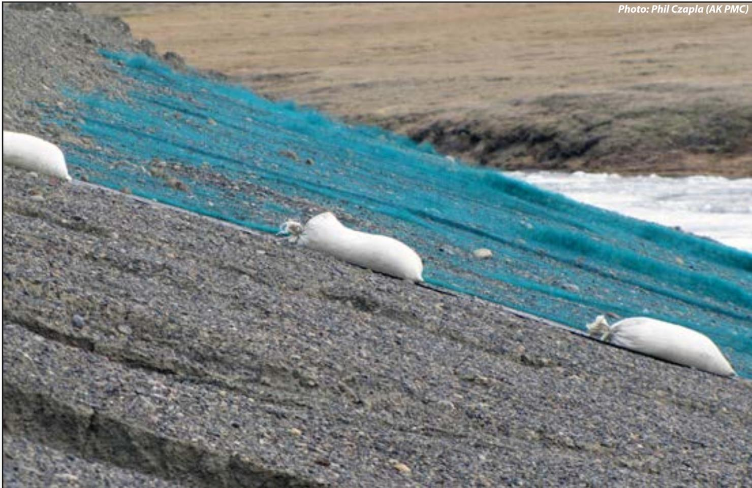
Geo-textile fabric armoring protects a constructed slope from wind and water erosion.
