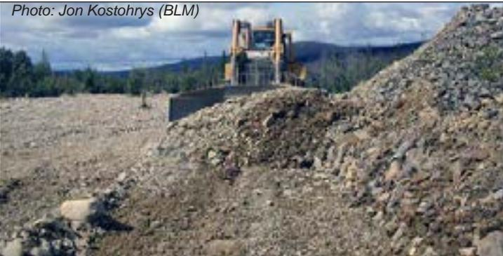
After filling the ponds, the bulldozer then graded the floodplain as flat as possible.
