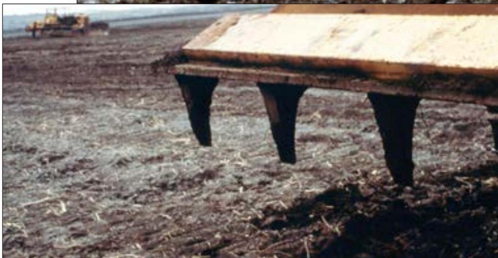
Deep scarification of the soil surface can be accomplished using a grader with a 'ripper shanks' tool bar.
