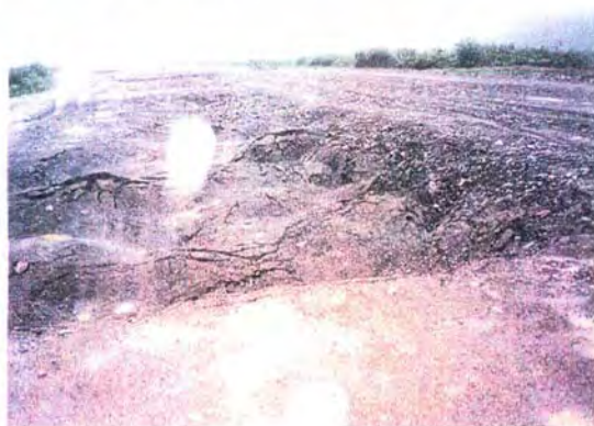
Mileposts 172 - 172.2. After corrosion dig in 1992 - workpad is subsiding.
