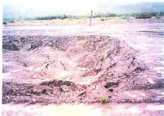
Mileposts 172 - 172.2. After corrosion dig in 1992 - workpad is subsiding.
