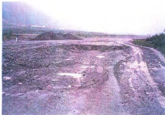
Mileposts 172 - 172.2. After corrosion dig in 1992 - workpad is subsiding.
