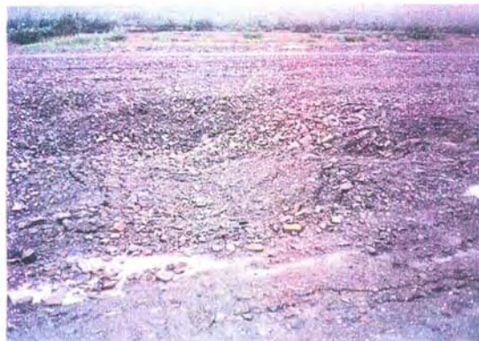
Mileposts 172 - 172.2. After corrosion dig in 1992 - workpad is subsiding.
