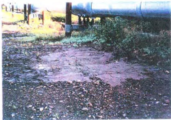
Creek crossing between Mileposts 416 and 417 should be monitored. Thermal erosion occurring upstream.
