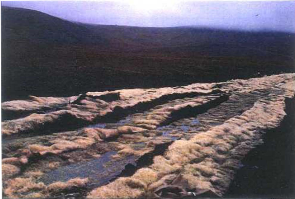
Figure 7. Trail after placement of Excelsior mat.
